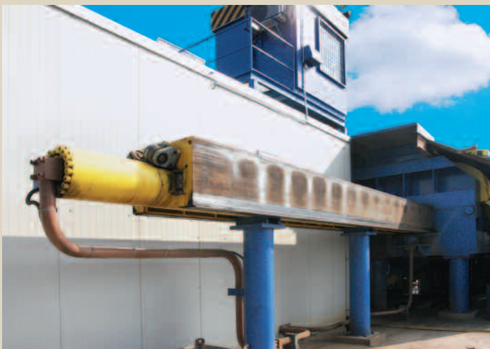
The pusher's hydraulic drive
